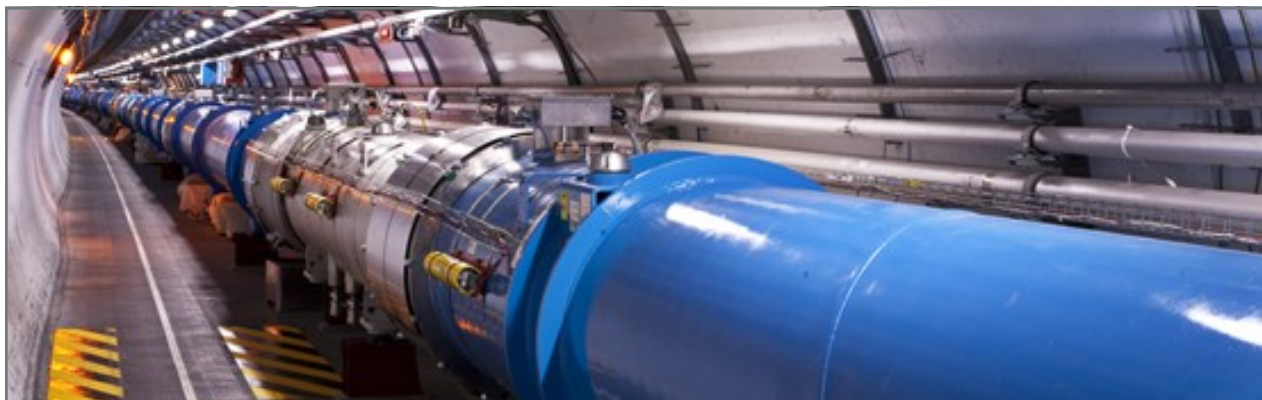
Figure 1. Views of the LHC Tunnel, Sectors 3 and 4
