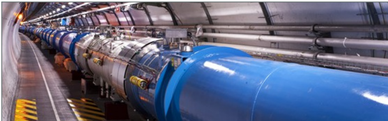
Figure 1. Views of the LHC Tunnel, Sectors 3 and 4
